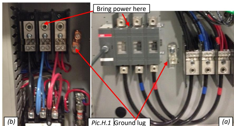
three-phase – see Pic.) are connected to the equipment – refer to the main label and submittal documentation.
