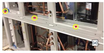
o locate the plastic covers/plugs at the front (a) and back (b) of the dehumidifier and pop them open to access screws;
