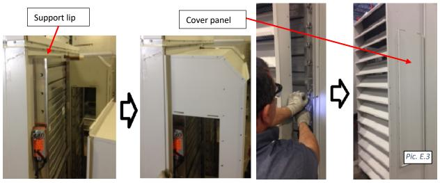
Outdoor AND Indoor Dehumidifier - Field-installed OA (outdoor air intake) Filter Rack Installation If the Outdoor Air intake (OA) filter rack is shipped separately, it should be attached to respective opening/damper once dehumidifier is installed. *This may apply to both, indoor and outdoor installed dehumidifiers.*
