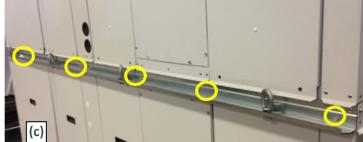
Remove as needed the lifting eye-hooks to allow for doors removal.
